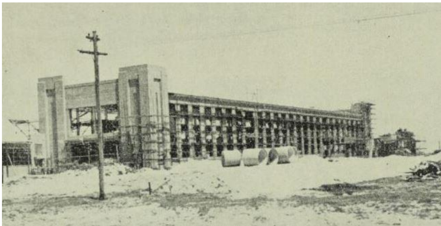
Figure 17 – Undated. Construction of the warehouse building.
