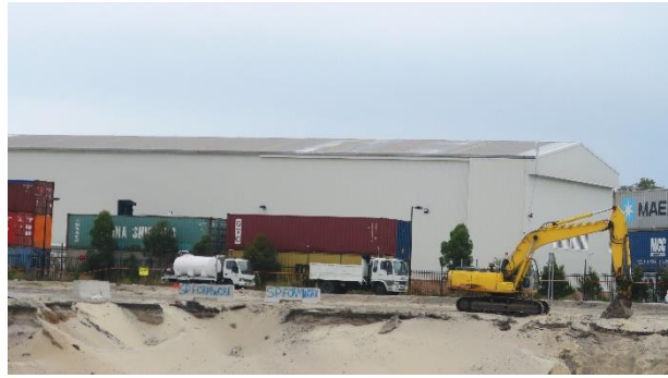
Picture 32 – Existing presentation to the south west.
