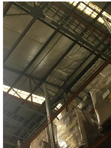
Picture 34 – Original roof structure.
